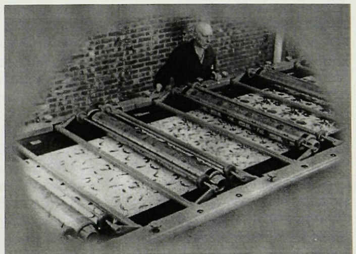
Fig. 5. Peter Zimmer's RSDM operating at van Vlissingen.
